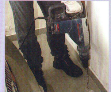
Concrete slabs have to be drilled.
