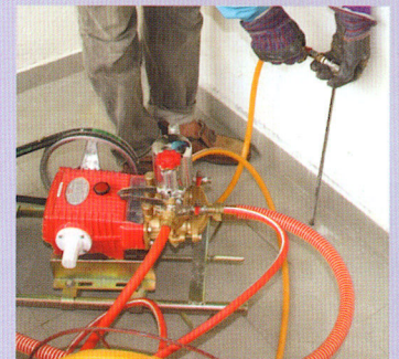
Premise 200 SC injected through slab. Each hole is filled with 5 liters solution.
