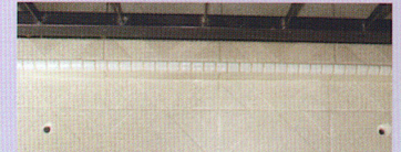
Holes are drilled at a distance of 50 cm.
